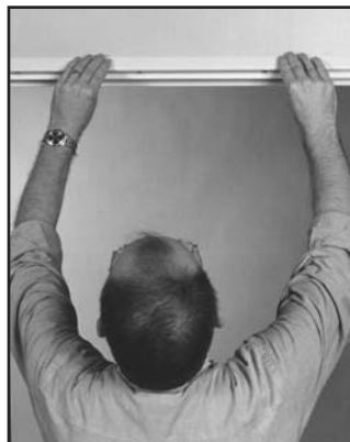
7 Snap on header casing.
