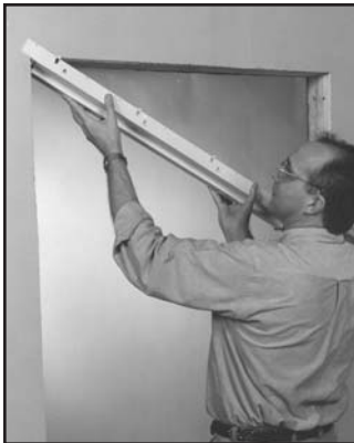
1 Set header over wall section.
