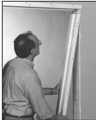
2 Set hinge jamb over wall section.
