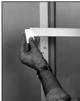
6 Slide corner backing angles into header casing.
