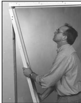
3 Set strike jamb over wall section.
