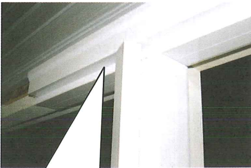
Cut the mull cap to the proper length. It goes from the brickmould down to the sill. The mull cap snaps onto the locking points of the jamb cover the same way the brickmould snaps on.
