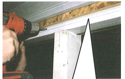
Screw the jamb cover between the two locking points on the jamb cover with the screws supplied in this kit.
