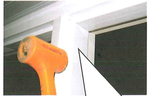
NOTE: Use a rubber hammer when applying nosing. Only tap on the corner of the nosing, if you tap on the center of the nosing it will dent.
