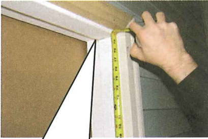
Measure from the inside of the header down to the sill to get the proper jamb cover dimensions for the mull post clad.
