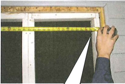
Measure to the inside of the vertical at the header.
